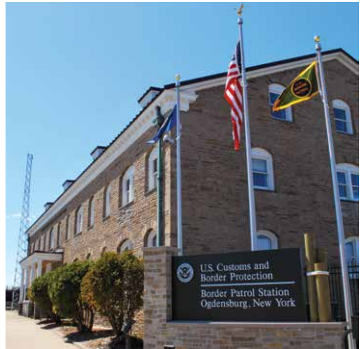
NKB provided A/E services for the historically significant Border Patrol Station in Ogdensburg, New York, located on the St. Lawrence River. The project scope included the upgrade and renovation of the oldest building on the National Historic Register to accommodate current immigration processing standards and protocol.
