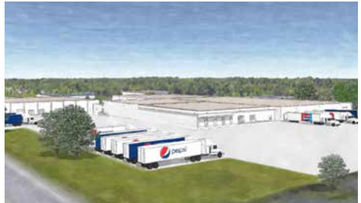
Westlake Development recently completed a $7.5 million redevelopment project for two of its tenants, including Pepsi.
