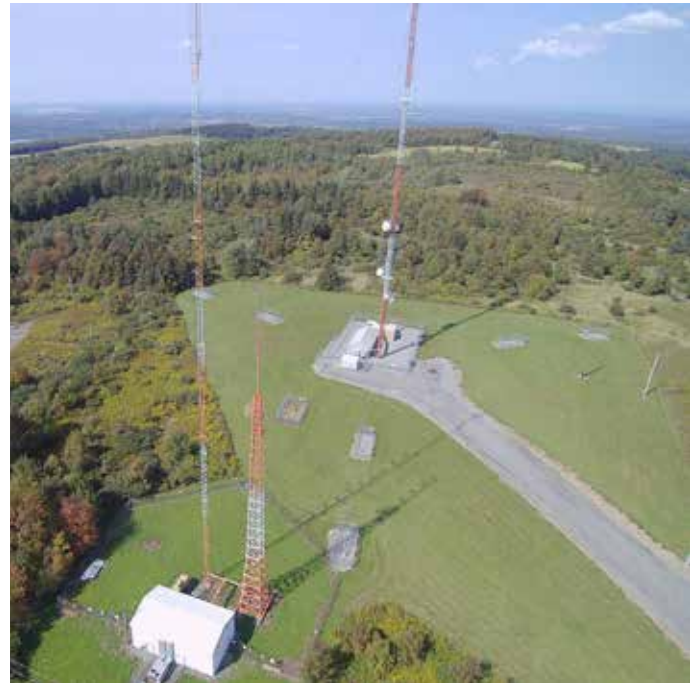
United Radio's tower inspection in Onondaga County.
