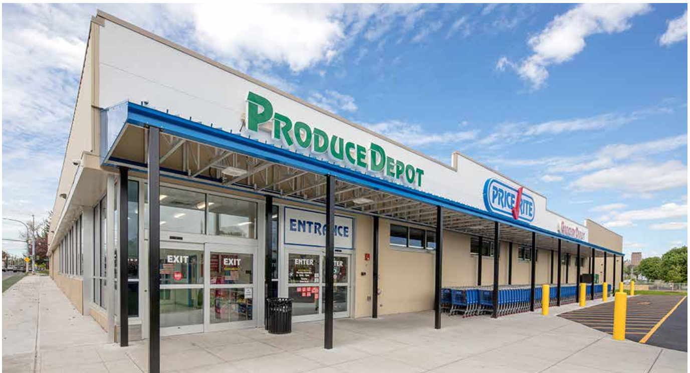
The new Price Rite store on South Avenue in Syracuse serves as model for inclusive development. Credit: VIP Structures.
