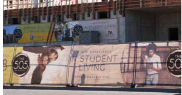
Three new student housing projects were under construction in 2017.
