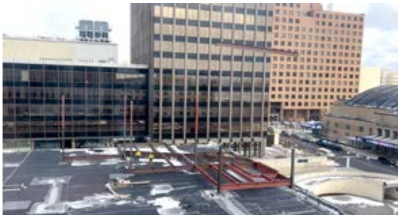
The Tech Garden construction underway, spring 2024. Credit: TangoSquared.
