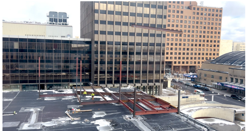
The Tech Garden construction underway, spring 2024. Credit: TangoSquared.
