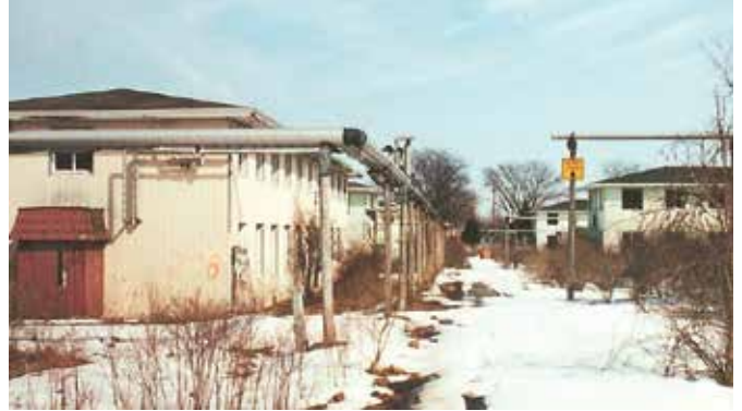
One of numerous military buildings, including exterior steam pipes for heating that was demolished at Hancock Airpark.
