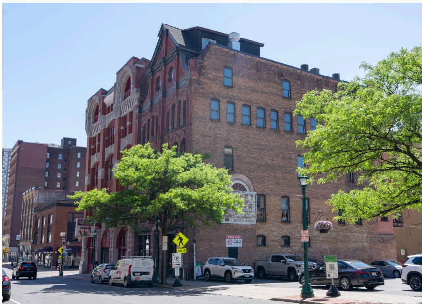
Copurpose office building at 316 S. Clinton Street.
